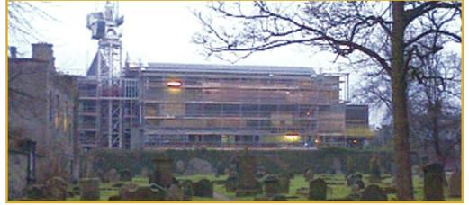
*Continued from page 1:* The art gallery spaces are in the process of having their steel framed roofs constructed and the metal bridges, which link the two halves of the building, will be installed soon. Sandstone cladding is being installed on the west elevation, and the restored façade of the former bank building on Abbot Street has been stripped of its scaffolding and is looking great after its repairs and clean up.
